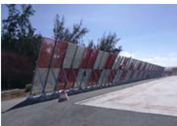
Picture 26. Blast fence. Gran Canaria Airport
